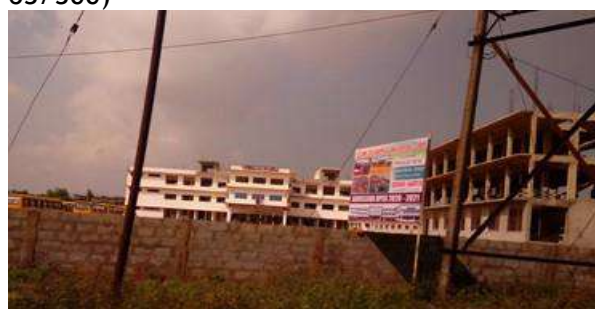
St. Joseph Higher Secondary School at km 64/600
