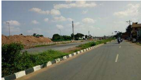
Section 2 start point at km 21/100 (NH 16)
