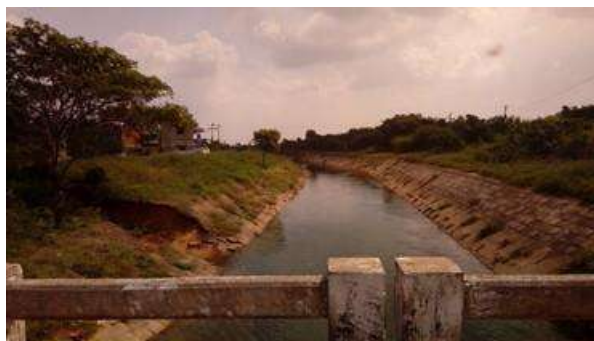
Krishna Water Channel crossing at km 53/700
