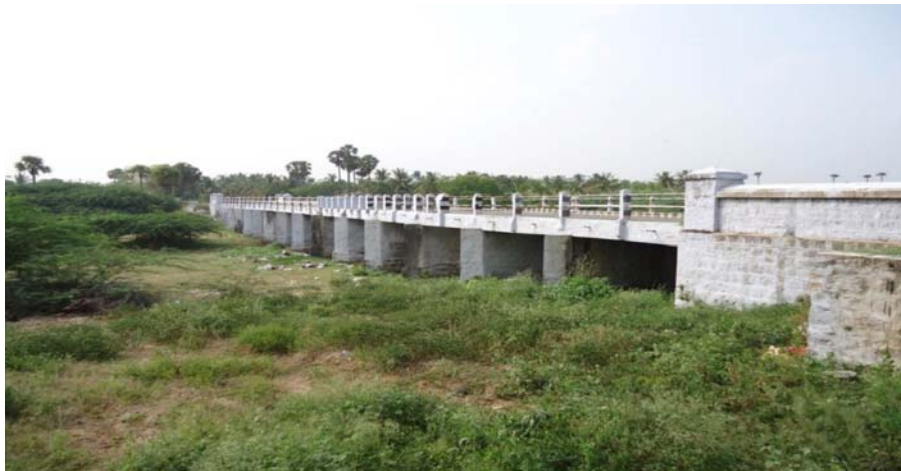
Major Bridge at Km 61+955
